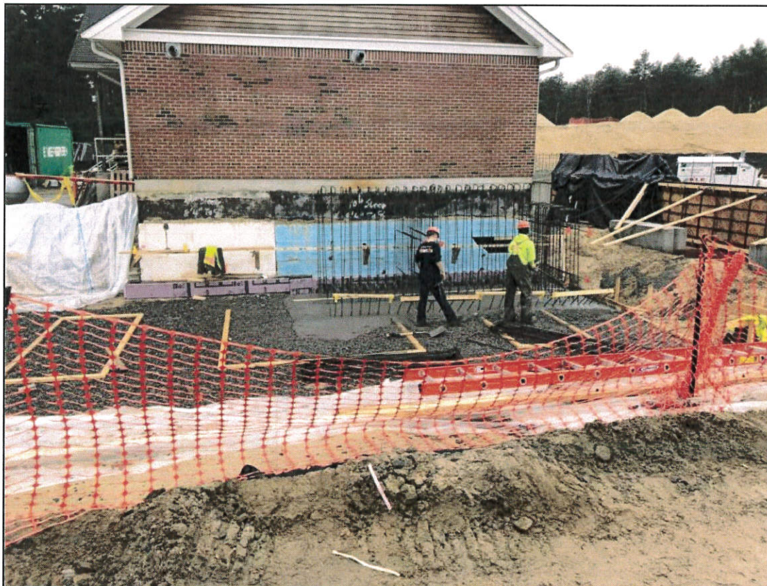
Picture 3: Maple Springs Water Purification Facility Construction.
